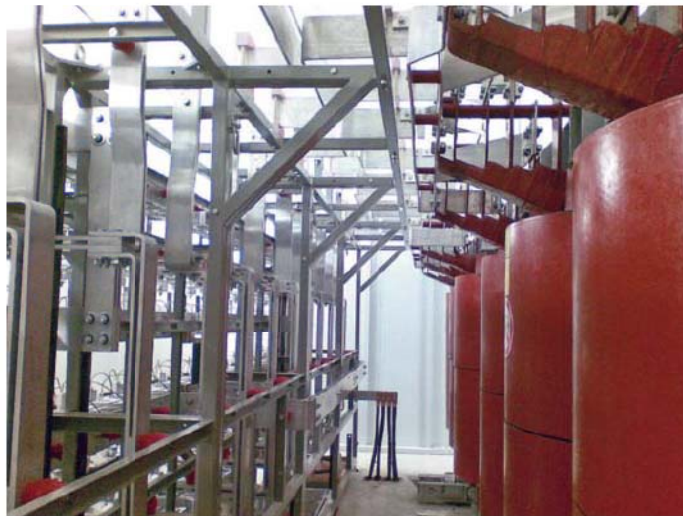
RAILWAY application 6.6MW 1500V 24 pulses Complete rectifier group: rectifier + transformers including bus bar connections among them
