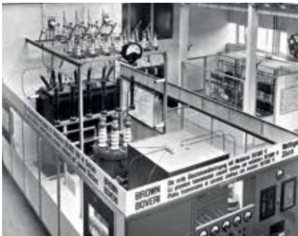
1939 First HVDC transmission line (pilot installation) Wettingen – Zurich, Switzerland
