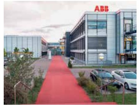
— 2010 Inauguration of expanded production facility at ABB Semiconductors in Lenzburg, Switzerland
